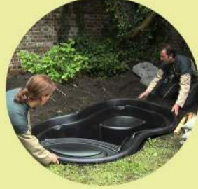
Step 3: Install The Pond Liner (Rigid And Rubber Liner)
