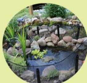
Step 9: Complete Building The Fence
